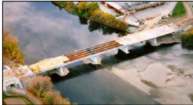
Figure 12.3: Aerial view of Joffre Bridge during construction.
