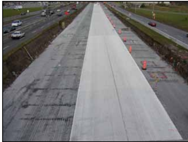
Figure 12.10: Continuous Reinforced Concrete Pavement with GFRP bars on Highway 40 East-Montreal.
