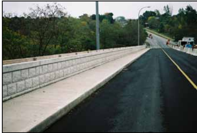
Figure 12.11: Deck Rehabilitation of Glendale Avenue Bridge.
