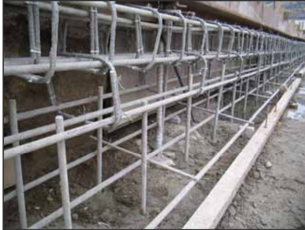
Figure 4.5: Inverted reinforced concrete T-beam reinforced with GFRP bars (courtesy of Pultrall Inc.).
