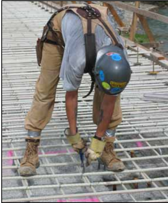
Figure 11.8: A construction worker stands on glass FRP bars while tying them together (courtesy Vector Construction Group).
