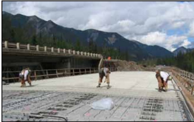
Figure 11.3: Placement of glass FRP bars in a bridge deck (courtesy Vector Construction Group).
