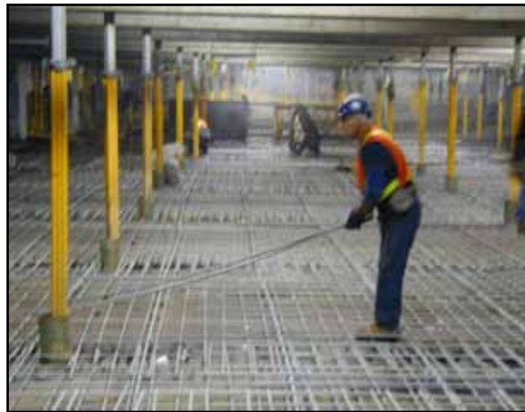
Figure 12.8: Placement of GFRP bars in Laurier Taché Parking Garage.
