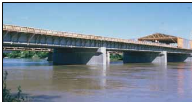
Figure 12.4: The Taylor Bridge, in Headingley, Manitoba, during construction.
