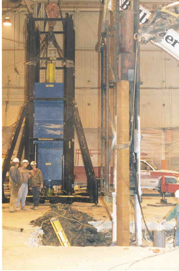
Figure 7-13. Statnamic Test Set-Up (courtesy of Applied Foundation Testing (AFT), Inc.).
