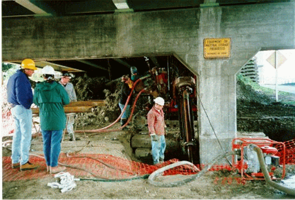
Figure 3-2. Low Headroom Micropile Installation.
